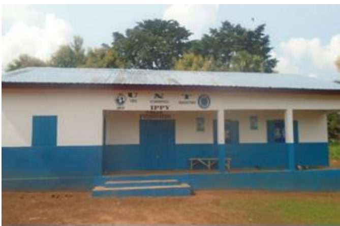
Figure 11 UNT building in Ippy built under the project
