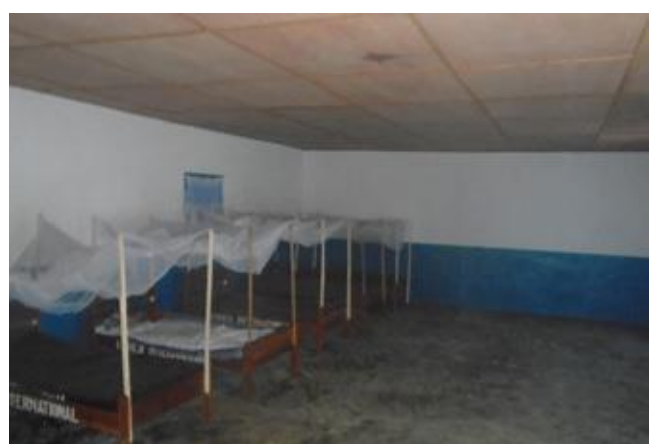
Figure 12 Ippy UNT building constructed as part of the project
