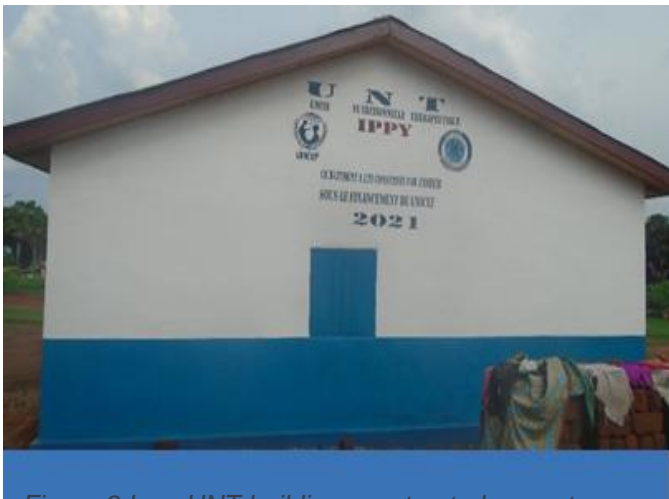
Figure 9 Ippy UNT building constructed as part of the project
